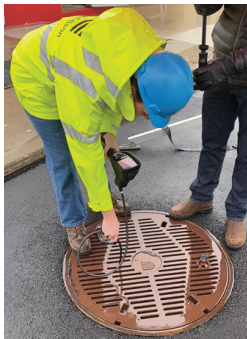
Figure 8.1 Inserting the probe into the test area.
