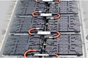
Battery charge/discharge test
