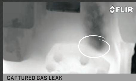
CAPTURED GAS LEAK
