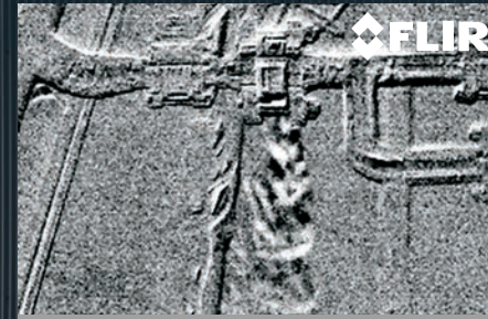
CO 2 LEAK - HSM IMAGE
