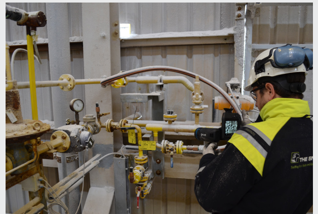
Philip Schraeyen and Jan Van Hout of The Sniffers using the GF77 camera to inspect for methane leaks
